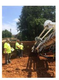
The college apparently came to the same conclusion, so they called Rembco to provide the design and drawings for a temporary soil nail wall. When our proposal was approved, we began construction and testing of a 26' soil nail wall. This isn't our first experience with similar construction at the University. In fact, Rembco first provided a similar shoring system for UT more than 30 years ago. Here's how we do it.
